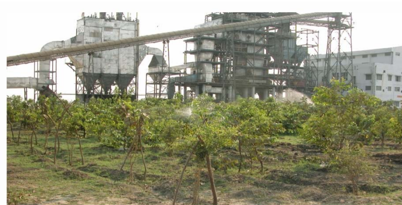
Part of the climate-offsetting investments is made in the biomass power plant Sri Balaji in the Indian state of Andhra Pradesh, a Gold Standard CDM-project.
